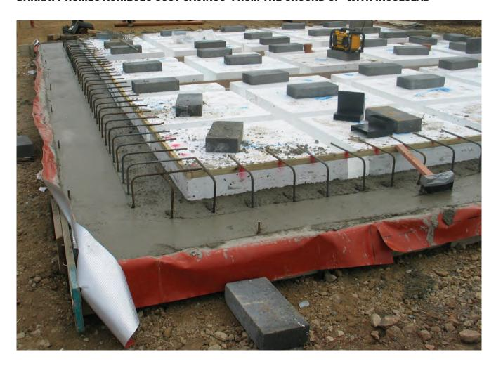
Barratt Homes has benefitted from both time and cost savings at 'The Elms', a new build development in Stockton on Tees, after replacing a traditional raft foundation structure with Insulslab.
